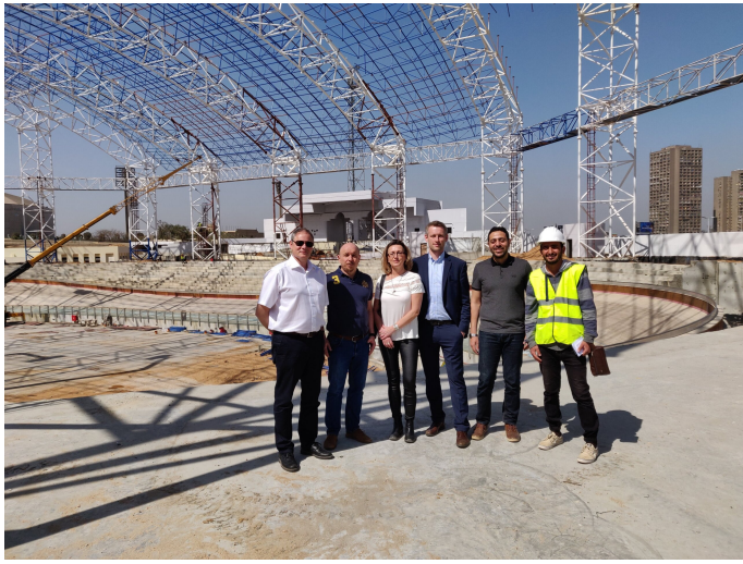
Representatives of the company Loesche GmbH on site in Egypt ©El-Fateh
